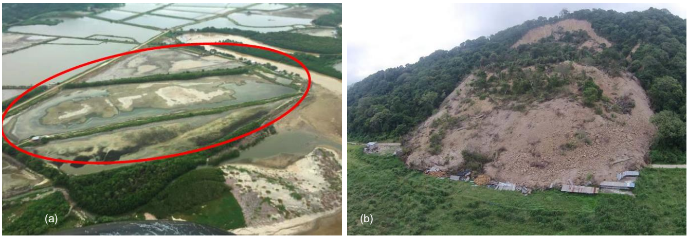
Fig. 5 – (a) Liquefaction evidence from GEER army helicopter flyover of Manabí coast, at Jama; (b) landslide on San Vicente-Canoa road. Source: GEER-ATC Report [1].
