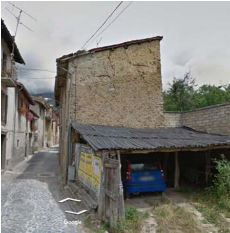
Fig. 4c – Horizontal arch mechanism involved upper part of a three floors rural building, Sommati village
