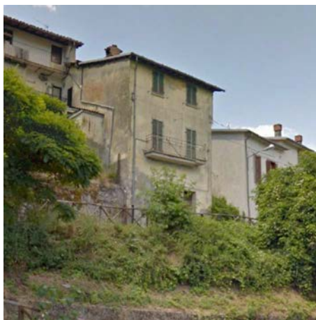
Fig.2d – A three floors slender building located on an elevated slope characterized by zero mechanism due to poor and disaggregated masonry, Saletta village
