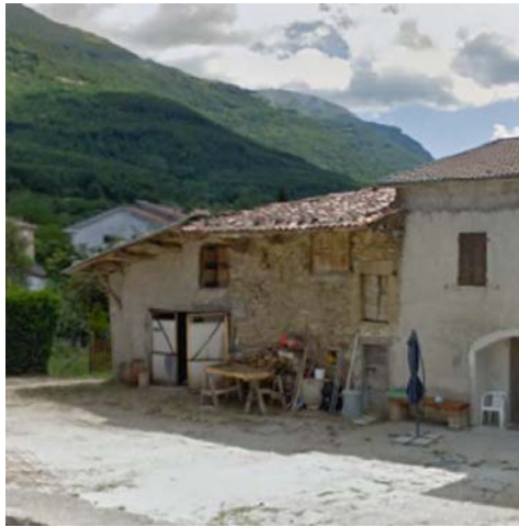
Fig.2e - Rural warehouse has collapsed by disaggregation. The less of maintenance get worse the originally main weakness: the poor quality of the masonry made of pebbles and mud mortar, San Lorenzo a Flaviano village
