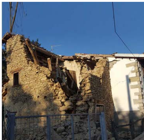
Fig. 4e – The rural building shows the corner collapse depends on the presence of quoins, on the layout of the opening and spanning direction of the roof, Faizzone village
