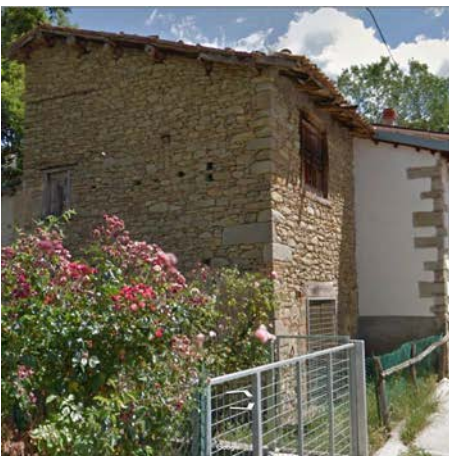
Fig. 4e – The rural building shows the corner collapse depends on the presence of quoins, on the layout of the opening and spanning direction of the roof, Faizzone village
