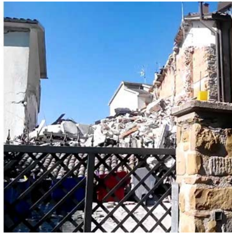
Fig.2c - Two terraced dwellings interlocked between higher buildings with stagger floors, collapsed by disaggregation, Saletta village
