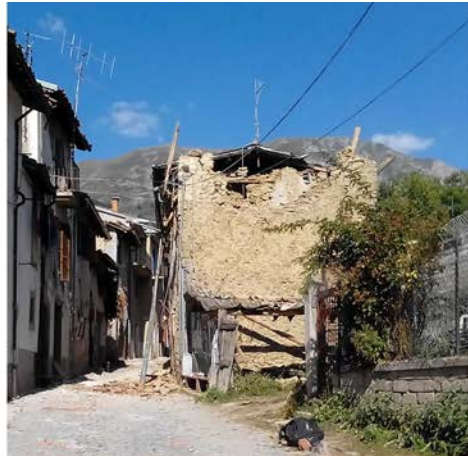
Fig. 4c – Horizontal arch mechanism involved upper part of a three floors rural building, Sommati village
