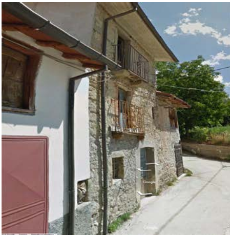
Fig. 4d- The building presents the activation of vertical arch mechanism due to lack of good connections between floor and masonry wall and to hammering of floor on rubble masonry, Faizzone village
