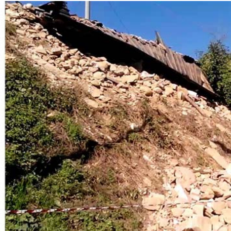
Fig. 2b- An isolated rural building subjected to a global collapse due to the disaggregation of masonry walls constituted by mud mortar and pebbles elements, Saletta village
