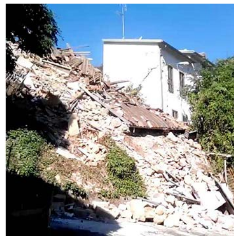
Fig.2d – A three floors slender building located on an elevated slope characterized by zero mechanism due to poor and disaggregated masonry, Saletta village
