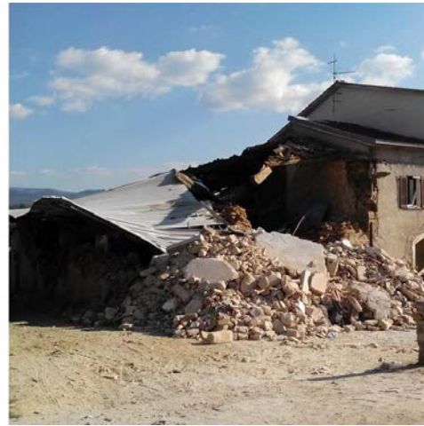
Fig.2e - Rural warehouse has collapsed by disaggregation. The less of maintenance get worse the originally main weakness: the poor quality of the masonry made of pebbles and mud mortar, San Lorenzo a Flaviano village
