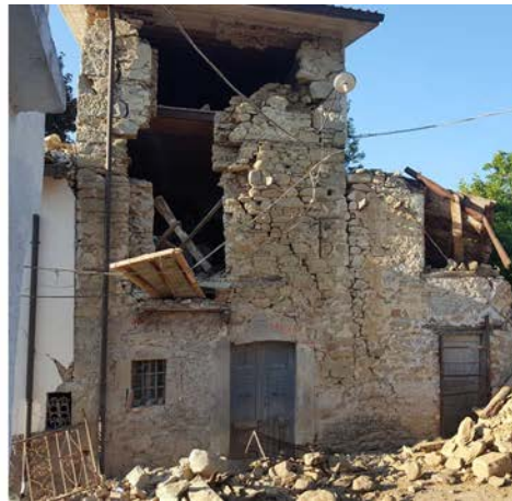
Fig. 4d- The building presents the activation of vertical arch mechanism due to lack of good connections between floor and masonry wall and to hammering of floor on rubble masonry, Faizzone village
