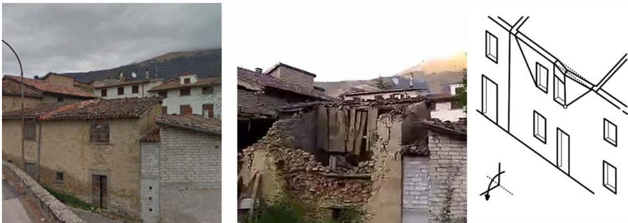
Fig. 4b- A rural interlocked building shows horizontal arch mechanism inducing the overturn of the façade and the separation of external leave of remaining wall, Sommati village
