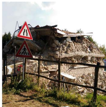
Fig. 3a/b – Two isolated dwelling due to stiff and heavy RC gable roof and floor sliding, have determined a global collapse of masonry structure, San Lorenzo a Flaviano village
