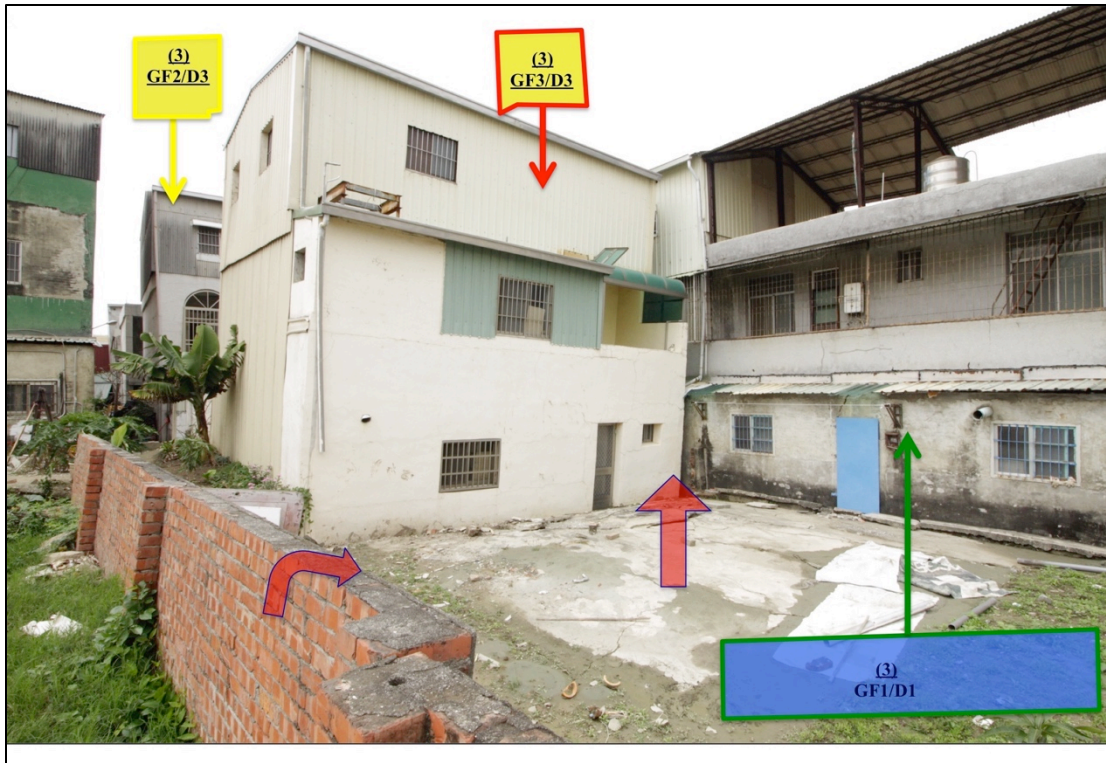
Fig. 9 – Example of mapping GF1 through GF3; demonstrating various structural damage states. (23.0254°, 120.2075°)
