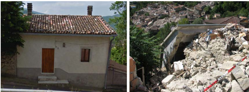
Fig.1 – Masonry building before and after the Central Italy earthquake, Pescara del Tronto.
