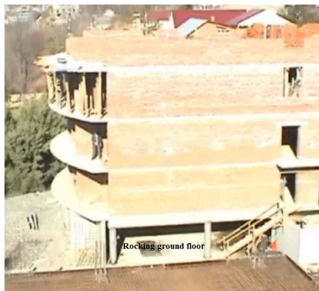
Fig. 1 – Full-scale dynamic tests of a rocking podium structure [1]
