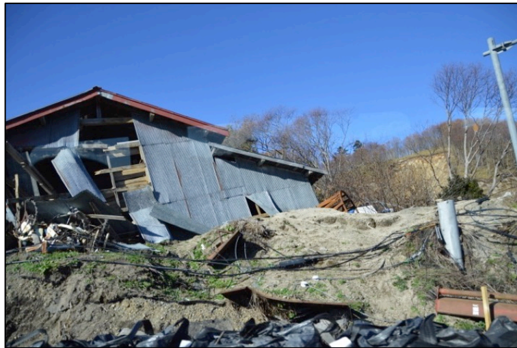
Fig. 3 – Damaged transmission and distribution telecom cables.
