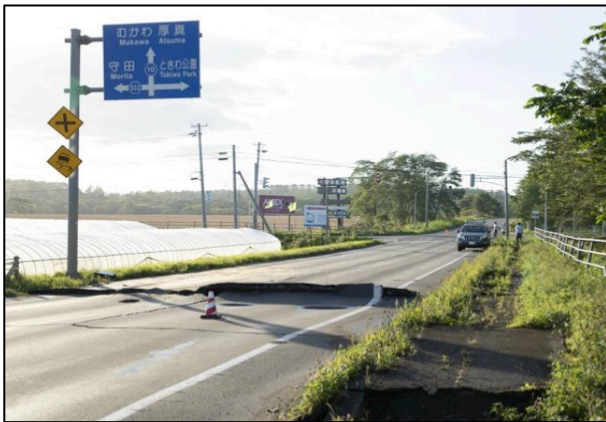
Fig. 10 – Surface compression failure (MLIT)
