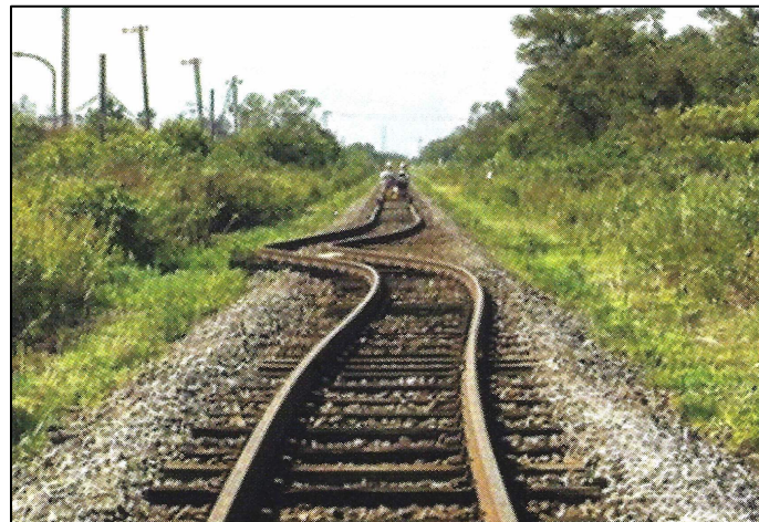
Fig. 13 – Twisted railway tracks (JR Hokkaido)
