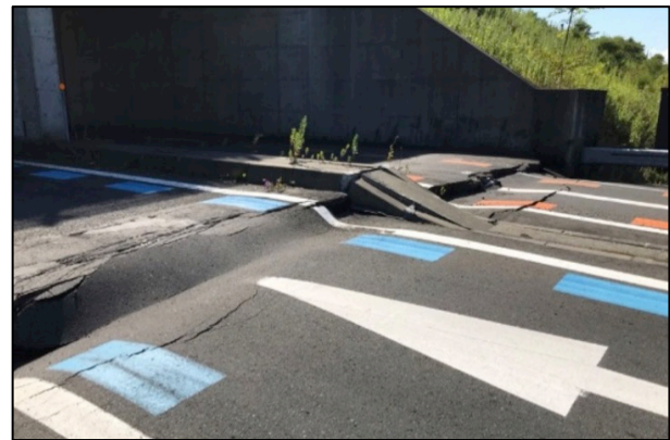
Fig. 11 – Surface compression close to the overpass (MLIT)
