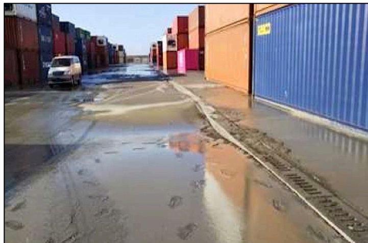
Fig. 15 – Liquefaction at a container storage area at the port (MLIT)
