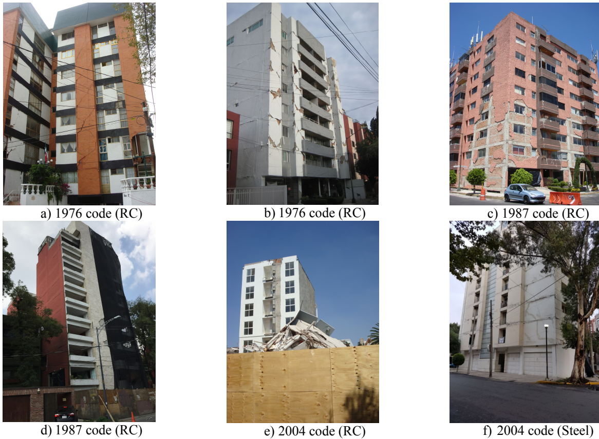
Fig. 7 – Some of the heavily damaged buildings design according to collapse prevention codes. Buildings shown in figures a) to d) have already been demolished. Front building in e) collapsed and the rear one was demolished. Building shown in f) was already retrofitted with concentric steel braces
