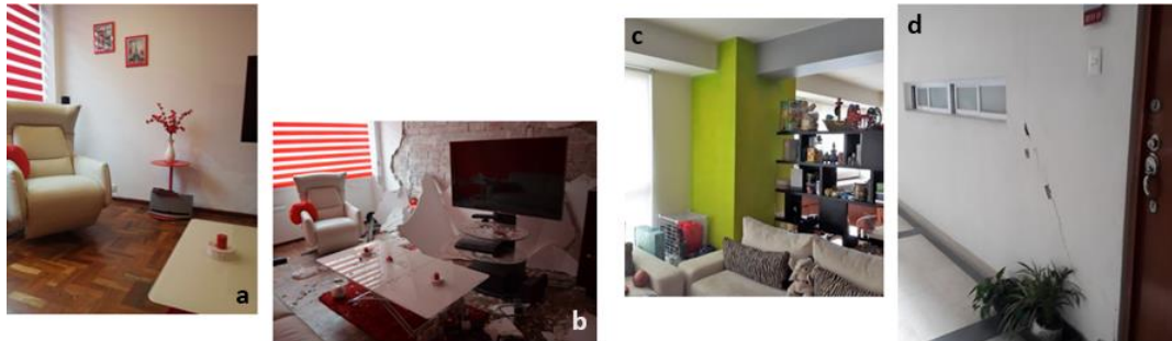
Fig. 16 – Damage to “non-structural” masonry walls. What should be acceptable
