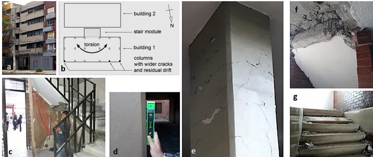
Fig. 8 – Torsion induced by stairs (a to e); extreme damages and obstruction of emergency exit (f, g)
