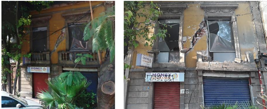
Fig. 12 – Pre-existing damage: Ago. 2014 (left) [4]; after 2017 earthquake (right)
