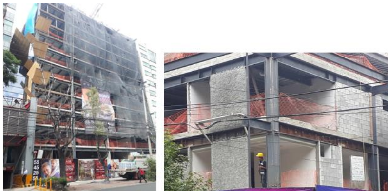
Fig. 15 – Buildings under construction – Left: too close to the adjacent buildings Right: with infills neither properly insulated nor connected to the structure
