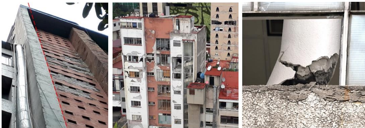
Fig. 5 – Damages due to pounding of adjacent buildings
