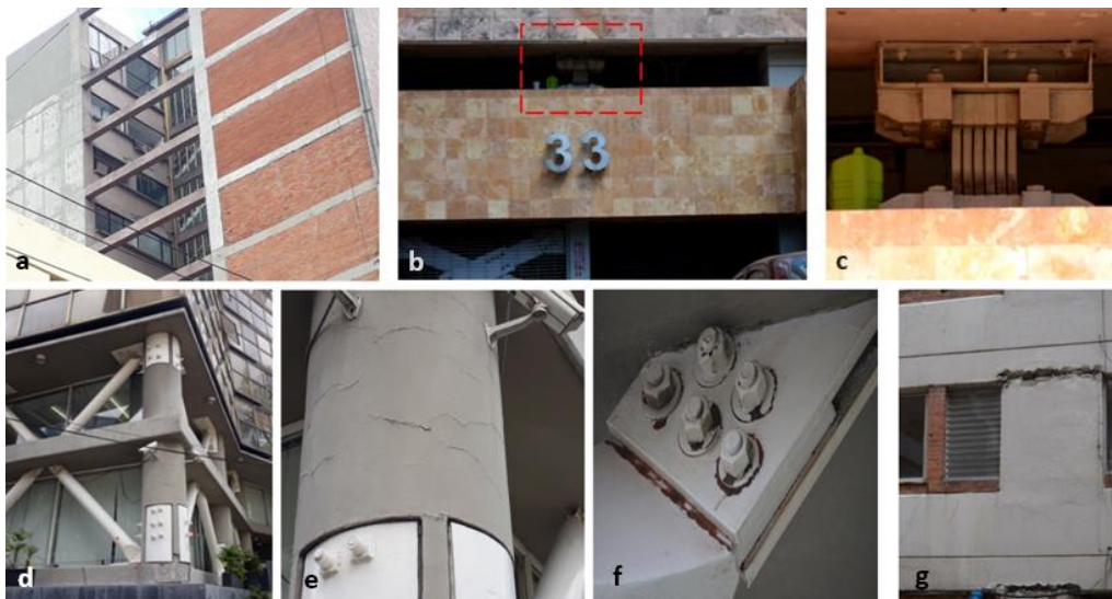
Fig. 11 – Examples of retrofitting techniques and their performance
