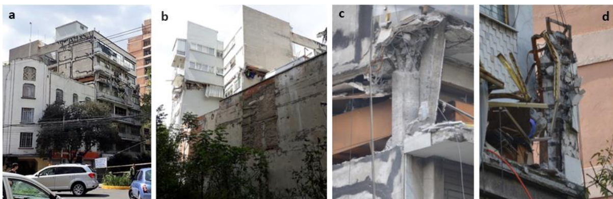
Fig. 13 – Collapse of a building due to the overlap of multiple factors
