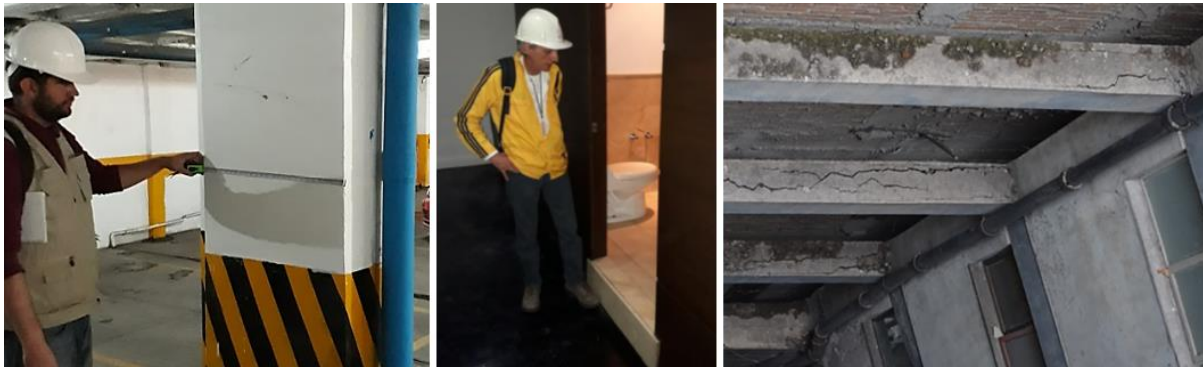
Fig. 6 – Deviations in dimensions; added overweight; corrosion damages
