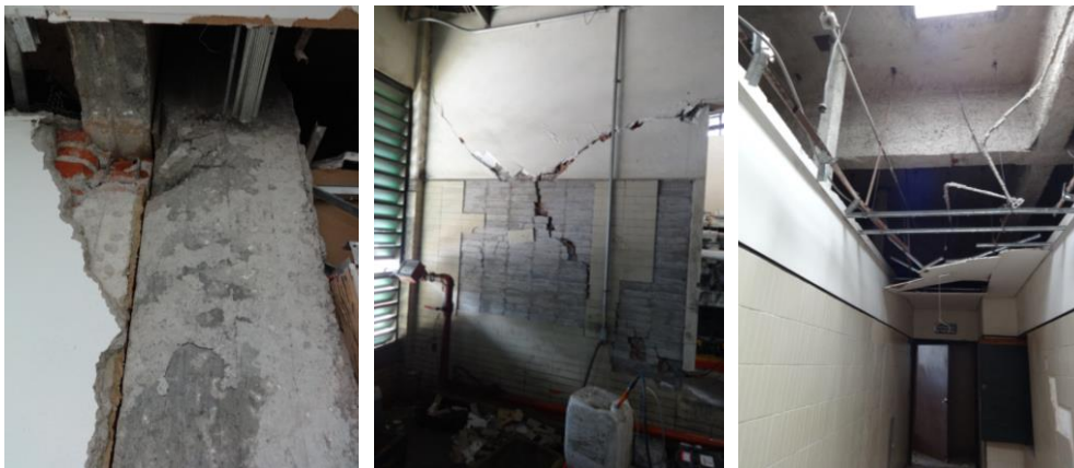
Fig. 5 – Typical structural and nonstructural damage due to S/19/2017/E in the IMSS Zonal General Hospital No. 7 at Cuautla, Morelos
