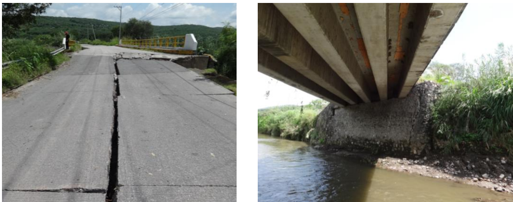
Fig. 6 – Typical structural and nonstructural damage due to S/19/2017/E in a bridge on the shortcut between Tlaltizapan and Tlaquiltenango, Morelos
