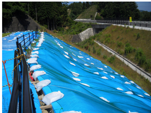
Fig. 1 An example of blue tarps (sheets) application to prevent successive failure of slopes
