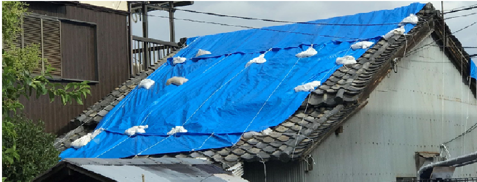
Fig. 2 An example of earthquake damaged roof covered by blue tarps (sheets)
