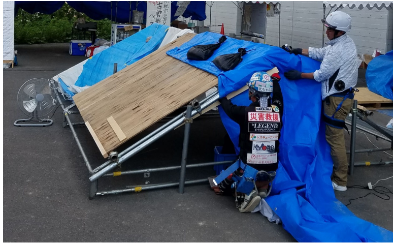
Fig.5 An example of workshop on how to install blue tarps for temporary restoration
