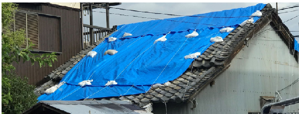
Fig. 1 An example of earthquake damaged roof covered by blue tarps (sheets)
