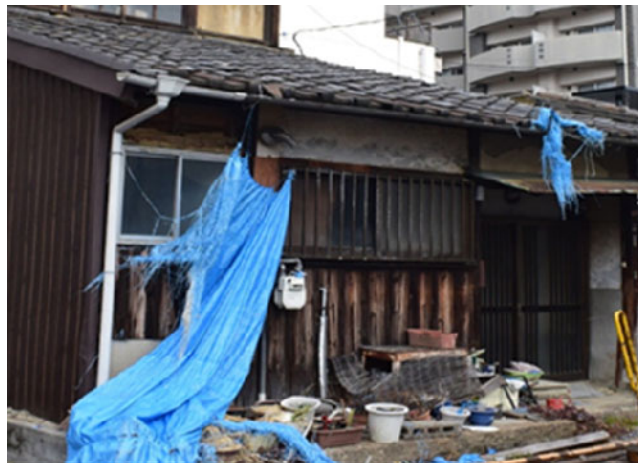
Fig. 3 An example of blue tarps (sheets) inappropriately used on a damaged house
