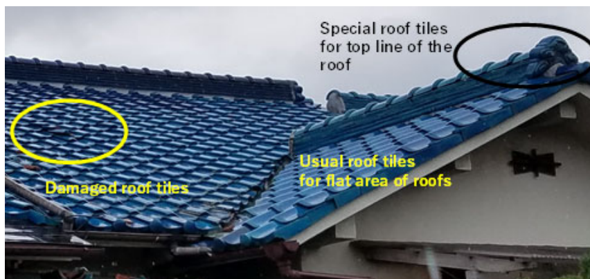
Fig. 4 An example of damaged roof and difference of roof tiles
