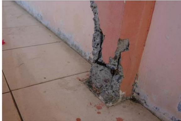
Figure 3. Concrete spalling at SNAN1 Lhoknga School
