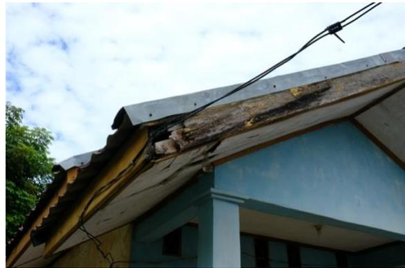
Figure 5. Rotting roof fascia and soffit timber boards, Kajhu
