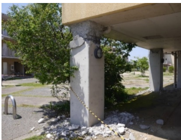
(a) Pillar viewed from the east
