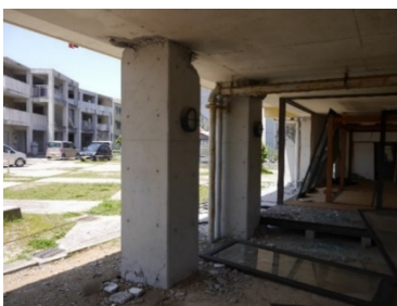
(a) Pillar viewed from the east
