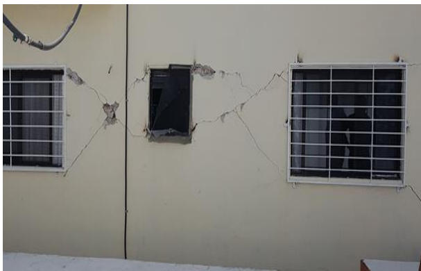
a) Rear facade
