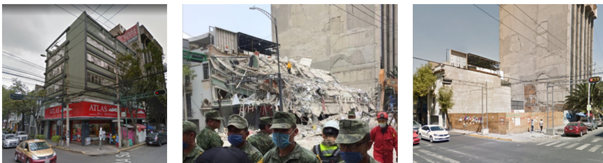
a) Before de 2017 earthquake b) during the 2017 earthquake c) After the 2017 earthquake
