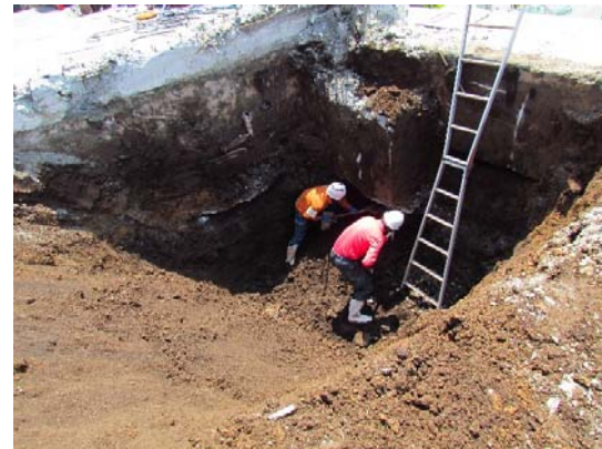
(b) Digging by manual
