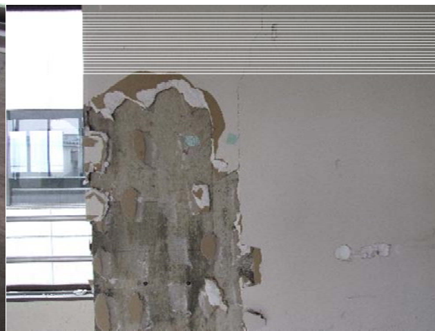
(b) RC wall with gypsum plaster board
