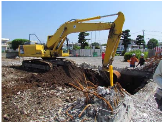
(a) Digging by excavator
