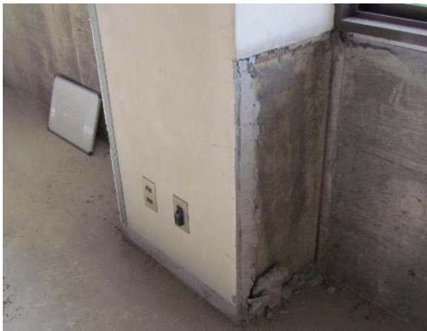
(a) RC column with mortar finishing
