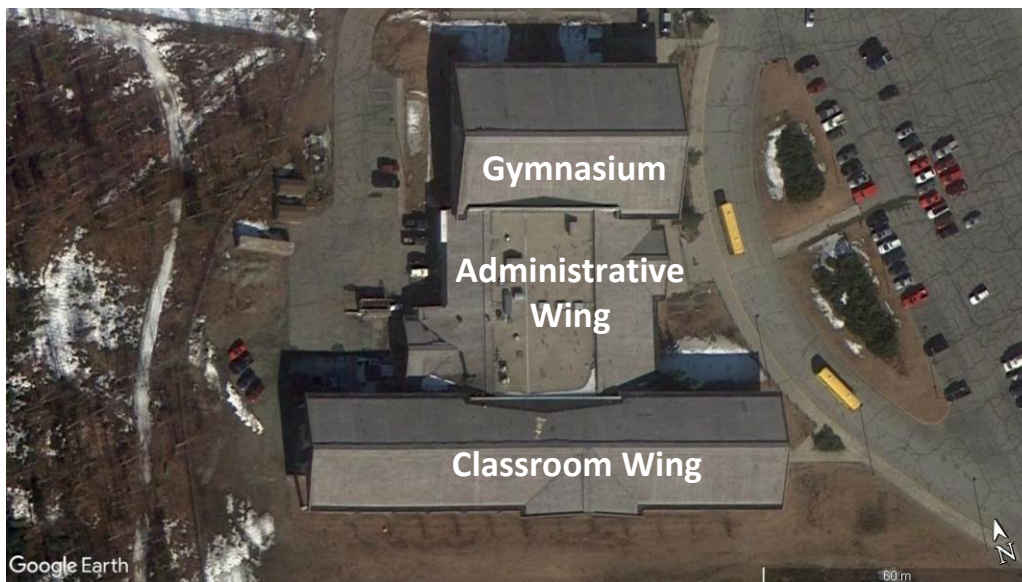
Figure 2 – Houston Middle School, showing the three main parts of the building. Imagery: Google Earth
