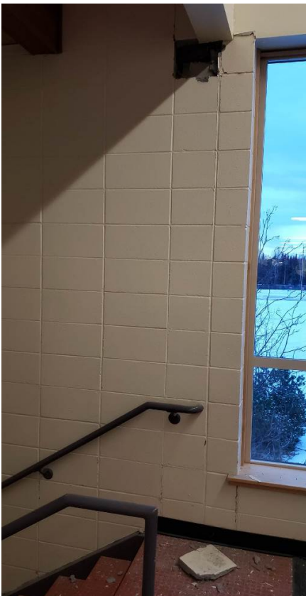
Figure 5 – Fallen block at stairs (left) and in hallway (right), Classroom Wing. The latter was dislodged by damage to the steel-girder to CMU wall connections shown in Figure 3. The classroom wing also suffered extensive damage to the suspended ceiling grid and tile, and many tiles fell. Photos: MSBSD
