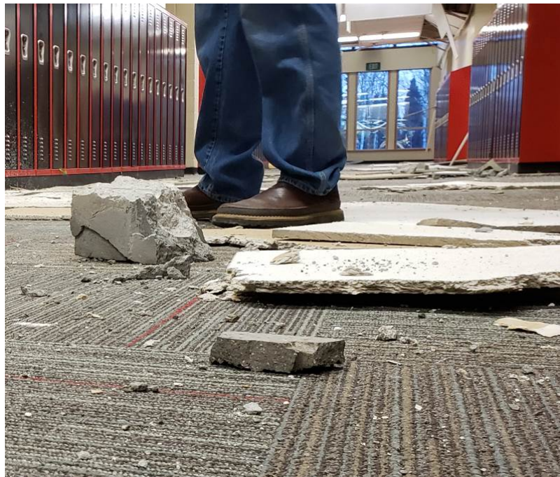
Figure 5 – Fallen block at stairs (left) and in hallway (right), Classroom Wing. The latter was dislodged by damage to the steel-girder to CMU wall connections shown in Figure 3. The classroom wing also suffered extensive damage to the suspended ceiling grid and tile, and many tiles fell. Photos: MSBSD
