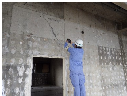
Photo 4 – Shear failure of wall girder above the opening of wall at Y3 frame of x-direction
