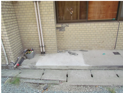
Photo 2 – Tile damaged at north Y4 frame spandrel wall
