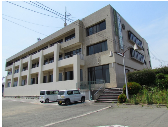
Photo 1 –Retrofitted R/C building damaged by the 2016 Kumamoto EQ
