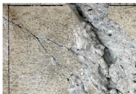
Photo 4 – Shear failure of wall girder above the opening of wall at Y3 frame of x-direction
