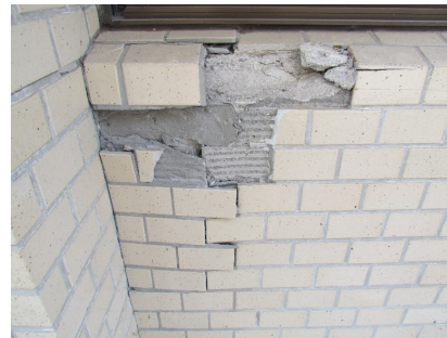
Photo 2 – Tile damaged at north Y4 frame spandrel wall
