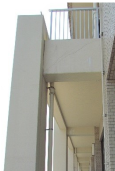
Photo 3 – Crack of connection beam between adding precast frame and existing R/C frame
