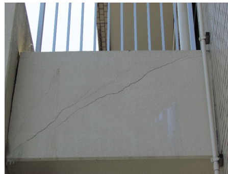
Photo 3 – Crack of connection beam between adding precast frame and existing R/C frame
