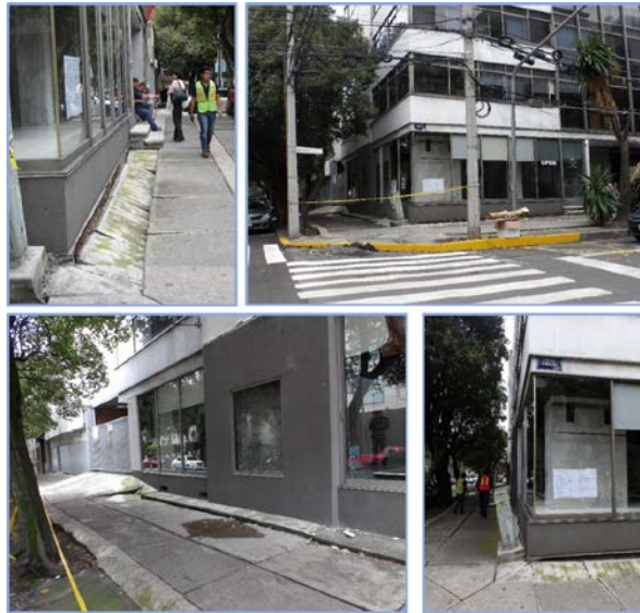
Fig. 12 – Tilting of buildings in Mexico City due to the September 19, 2017 earthquake and the related differential displacement affecting the building foundation. The structural components of the building were generally undamaged.
