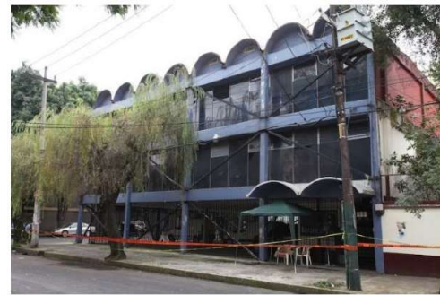
(b) Steel bracing of reinforced concrete commercial building
