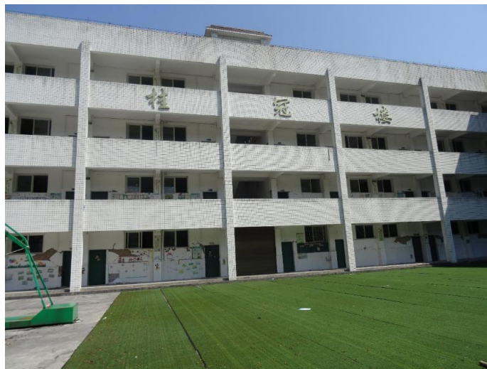
Fig. 12 –The frame structure school buildings without obvious damage during earthquake
