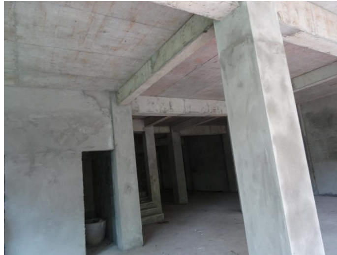
Fig. 11 –No damage in the earthquake of self-built frame structure buildings
