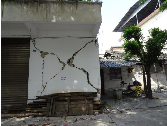
Fig. 8 – "X" cracks of brick concrete structure building in disaster area
