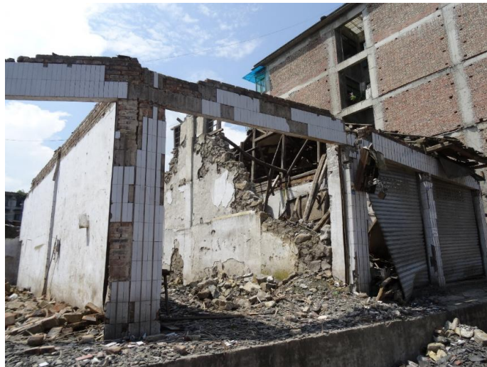
Fig. 7 – Destruction of brick and wood structure buildings in disaster area
