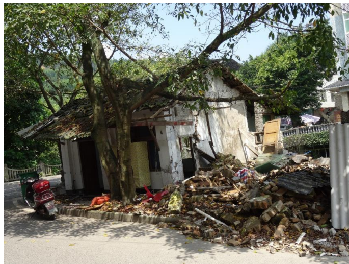
Fig. 5 – Collapse of brick wall and roof of brick wood structure buildings in disaster area
