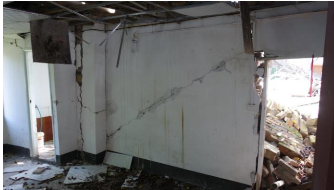
Fig. 6 – The brick and wood buildings with obvious cracks in the wall
