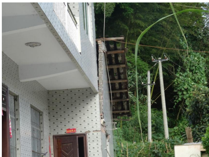
Fig. 10 –Displacement of brick concrete structure building wall in disaster area
