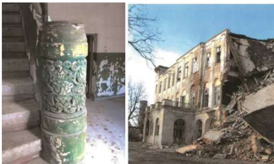
Fig. 4 – Left - Railing detail; Right - The posterior existence facade [12]
