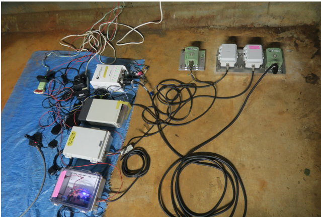
Fig. 5 – Settings of sensors at site TUN (Laser tunnel). An aluminum plate of 20mm thickness was fixed by anchoring the concrete floor of alcove, where is located at center of the laser tunnel, and the sensor was screwed on it. For sensors, anti-clockwise from right top, Titan in green and A352 in gray. For loggers, left top is Centaur and left bottom is the prototype for A352.
