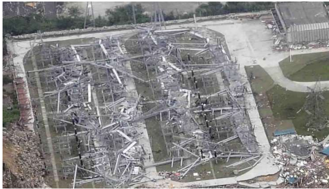
Fig. 1 Demolition of electrical substation in Wenchuan Earthquake
