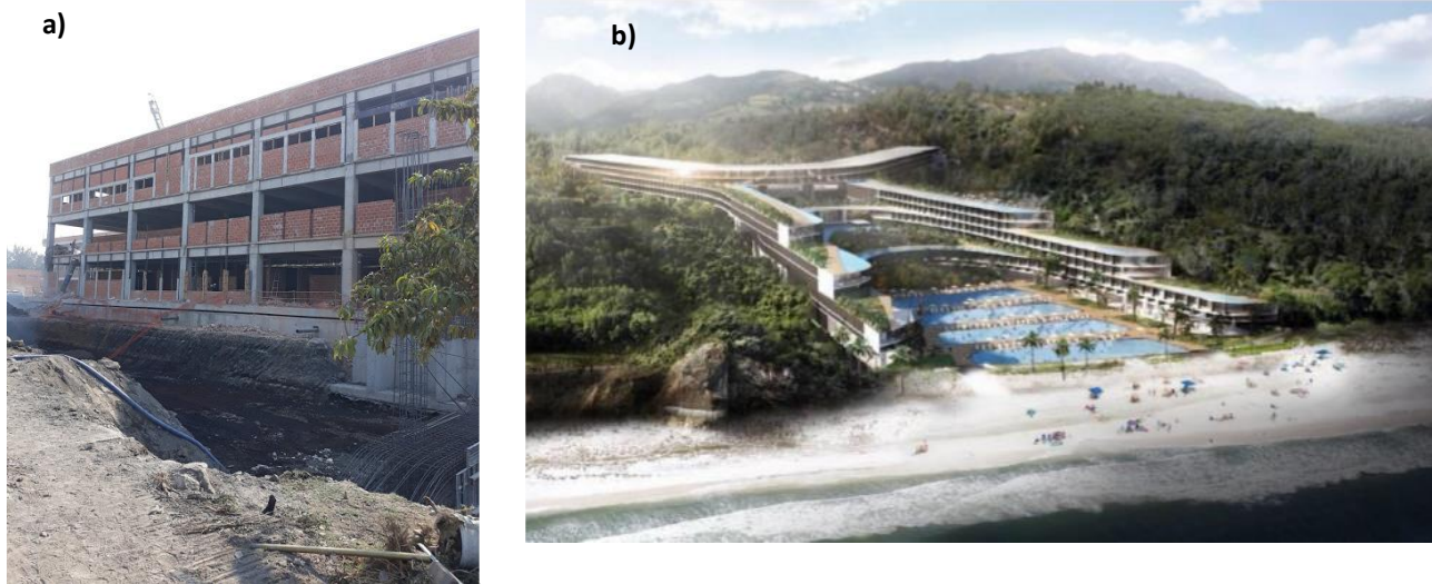
Fig. 7 – Base-isolated facilities: a) Hospital, Mexico City; b) Resort, Mexican Pacific Coast
