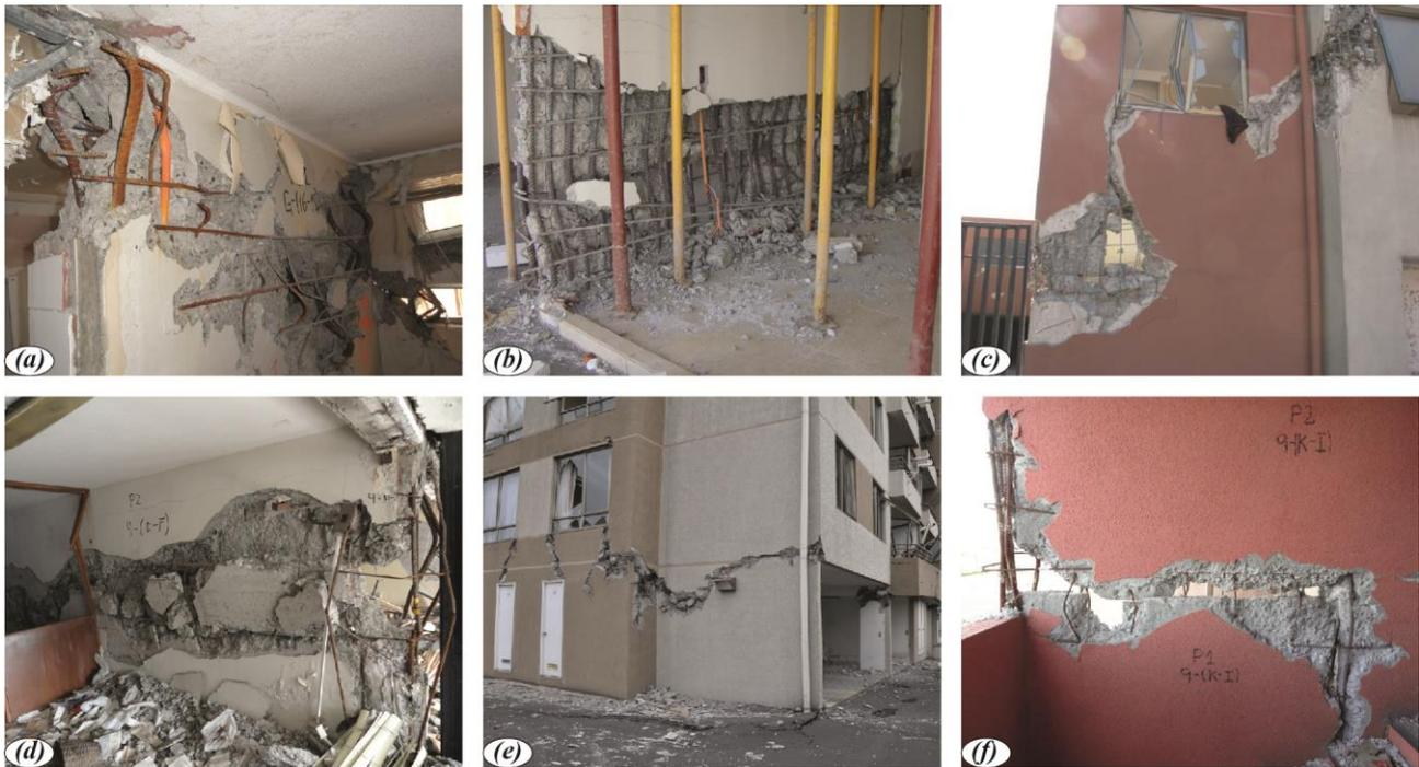
Fig. 1 – Examples of wall damage in buildings; (a) AA-1; (b) AH-2; (c) CM-3; (d) TL-4; (e) PR-6; and (f) RT-8; during the 2010 Chile earthquake [3].
