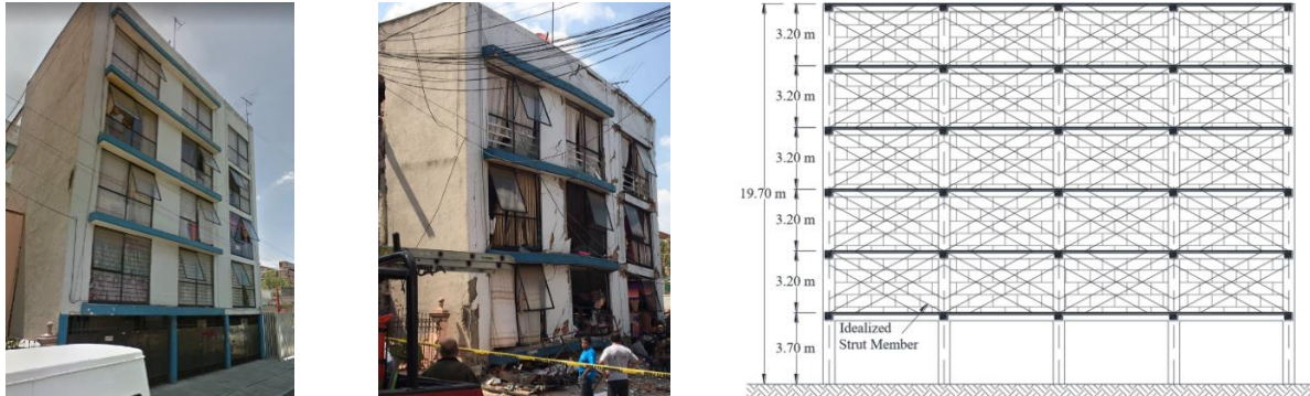
Fig. 1 – (a) Building with soft floor [15] and collapse [16], (b) Prototype building [17].
