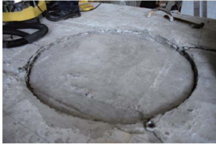
Fig. 10 – Sinking of top plate of specimen L3a.
