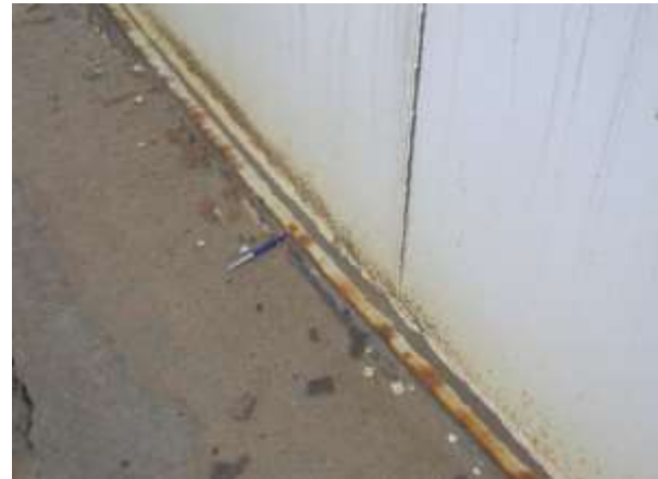
Fig. 7 – Response spectrum for horizontal displacements. Interplate subductive earthquake of Chile 2015, Illapel. Fig. 8 – Tank TK-201 with horizontal sliding, Tocopilla 2007.
