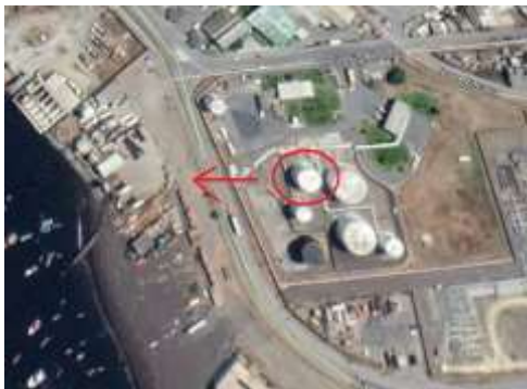
Fig. 11 - Gas storage tanks in Puerto San Vicente. El Maule 2010 earthquake. Red arrow indicates seismic directivity.
