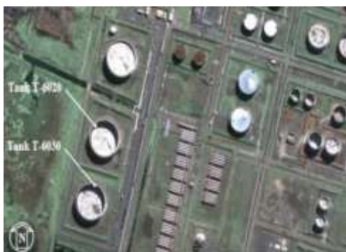
Fig. 13 - Oil storage tanks at the ENAP Bío Bío Refinery during the El Maule 2010 earthquake.
