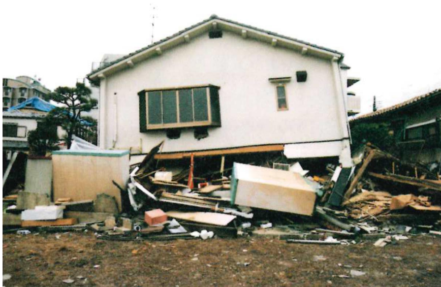
Fig.1 A wooden house damaged by story collapse on the first floor [1]
