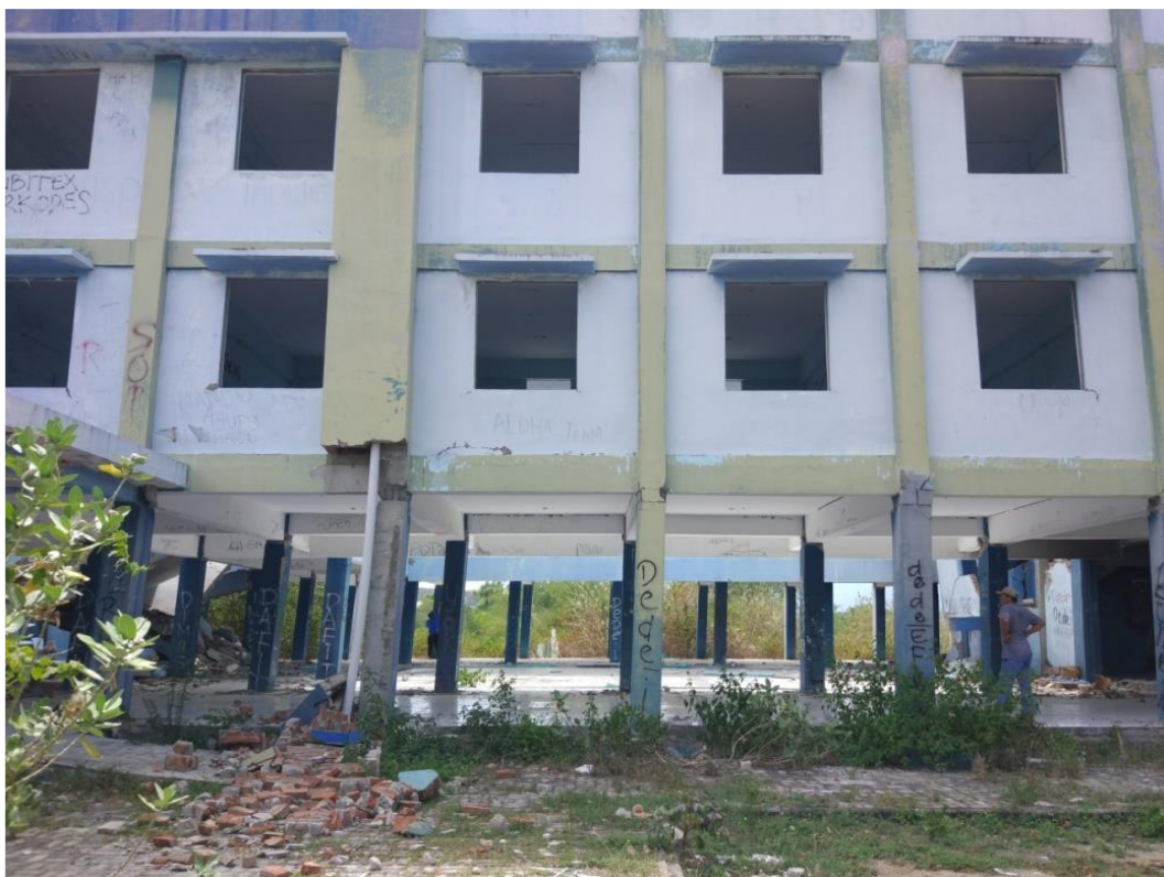
Fig. 3 – Front view of damage occurred on rental low-cost housing flat Univ. Tadulako
