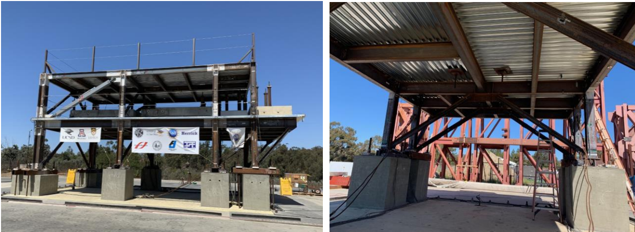
Fig. 12 – NHERI@UCSD Shake Table: (a) Phase 3 Test Specimen; (b) Composite Floor Deck Orientation.
