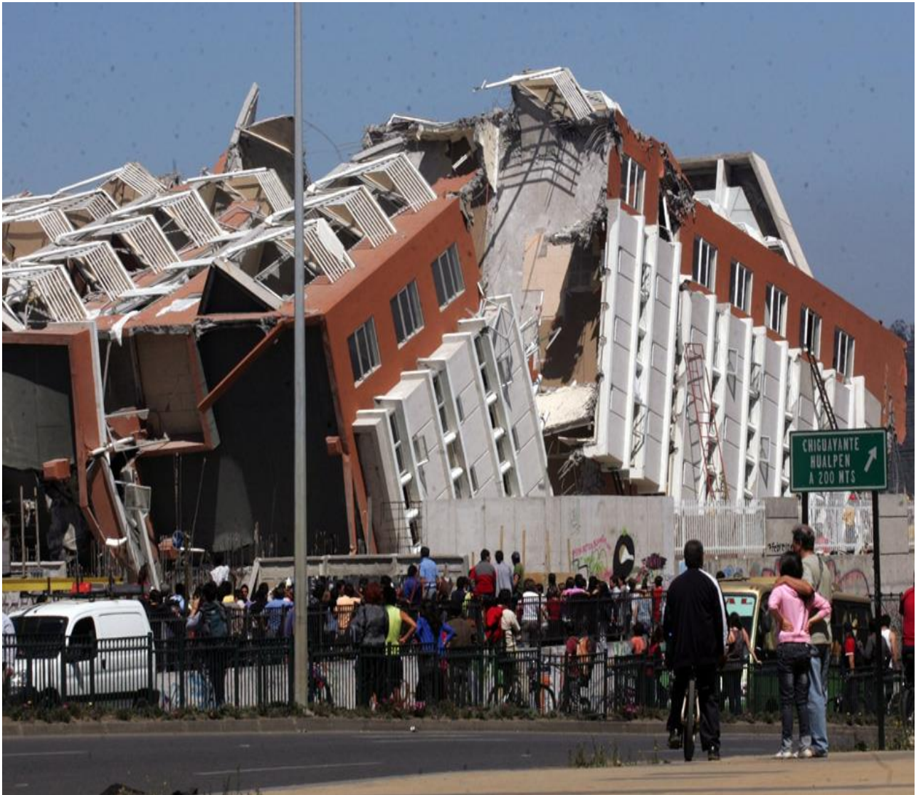
Fig.6 – Chilean Earthquake Damage
