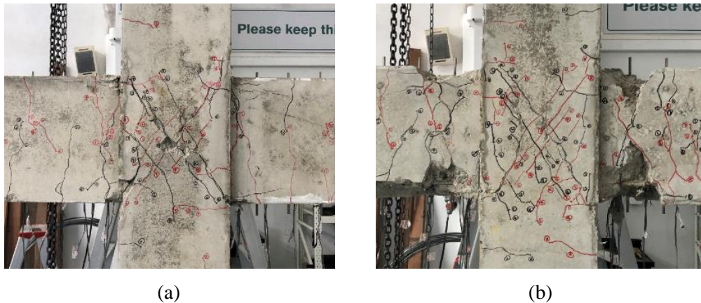
Fig. 7 – Crack patterns and failure modes of specimens (a) BCJ-S and (b) BCJ-D
