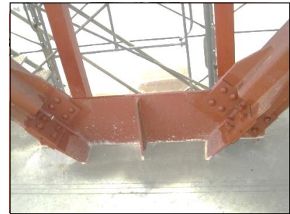
c) Joint of outer tube and frame
