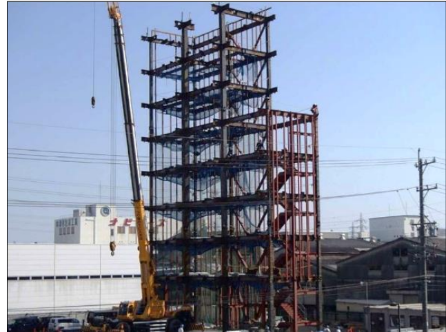
e) Construction status (full view)
