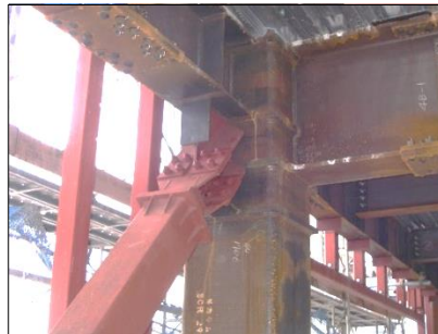
b) Joint of core and frame
