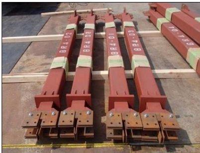
a) Shipment situation of brace
