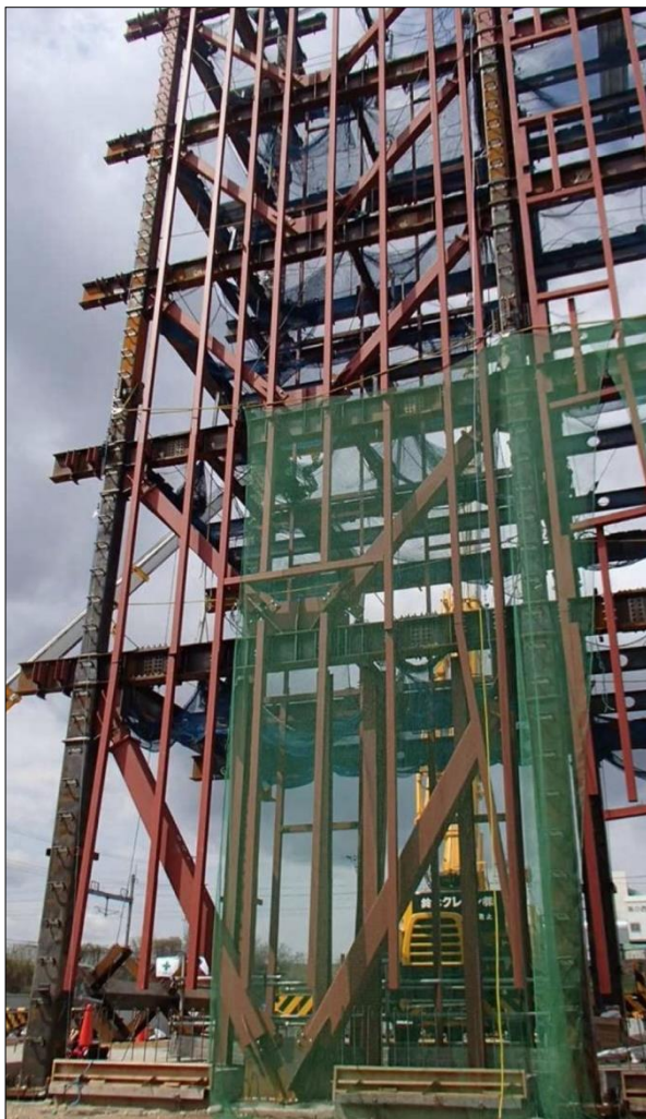
d) Construction status (full view)
