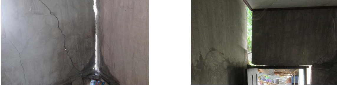
Fig. 8 – Separation of confining elements and masonry
