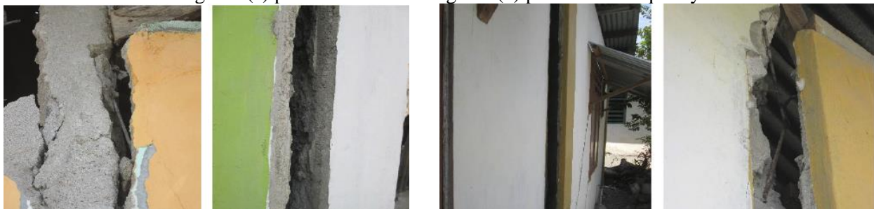
Fig. 7 – Splitting column due to poor concrete quality
