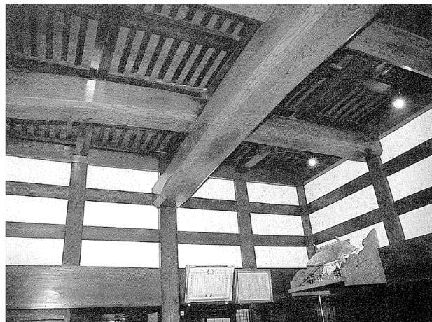
Fig. 1 – An example of the structure called “ Waku-no-uchi ” in a Japanese traditional timber house [1]
