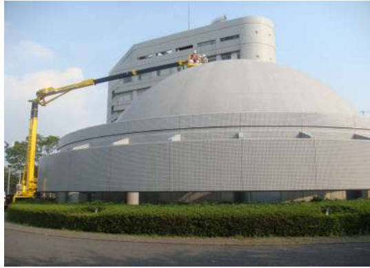
Photo 1–Spherical concrete shell in Chiba prefecture (Planetarium, Span:23.2m, Rise:8.11m, Positive Gaussian curvature)
