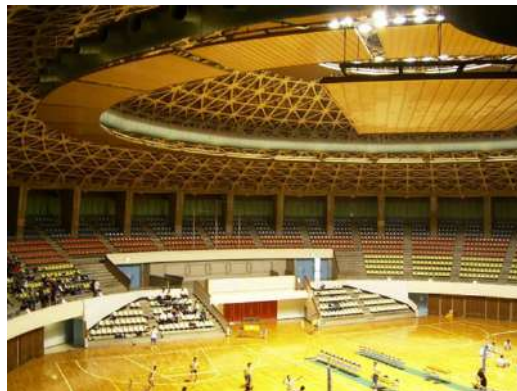
Photo 2–Conical steel framed shell in Chiba prefecture (Sports center, Span:68m, Zero Gaussian curvature)
