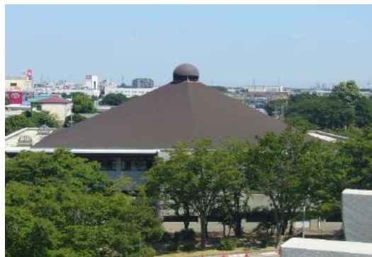
Photo 3–Hyperbolic paraboloidal steel framed shell in Chiba prefecture (Martial arts gymnasium, the Outside, 44m x 44m, Negative Gaussian curvature)
