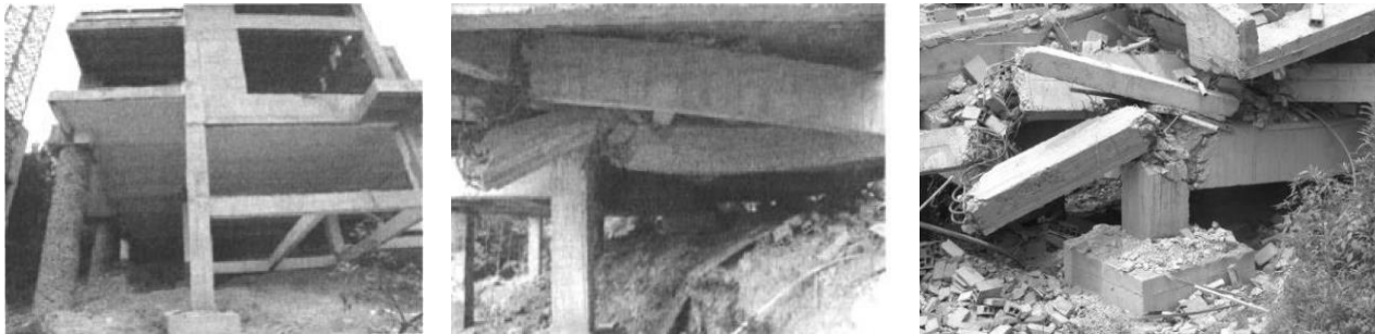
Fig. 1 – Seismic damage to stilted structures during the Wenchuan earthquake.
