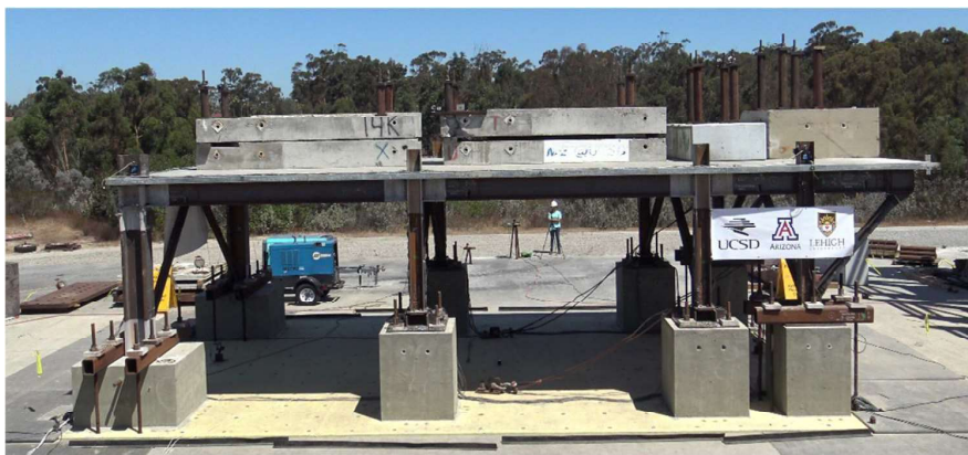
Fig. 3 –Phase 1 test frame
