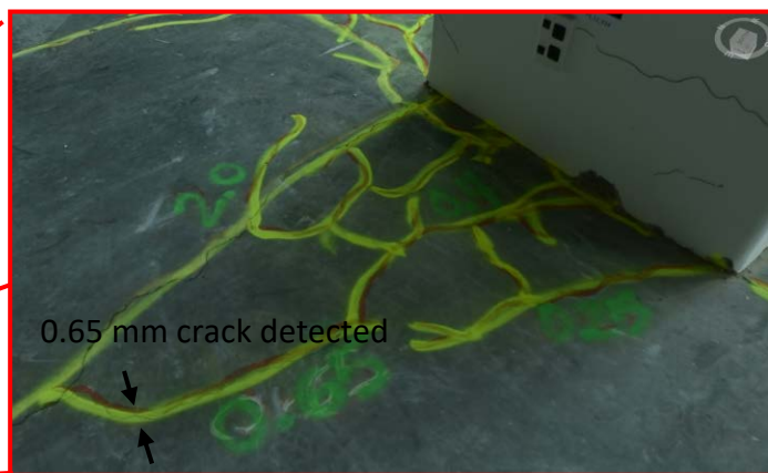
(f) Damage data collected using SFM
