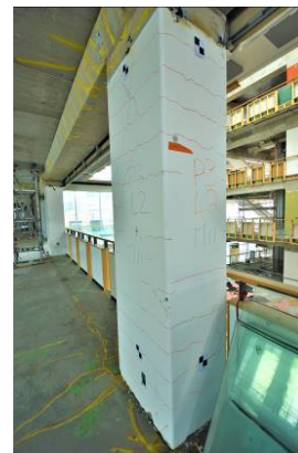
Fig. 2- Targets locations on top and bottom of each face of columns
