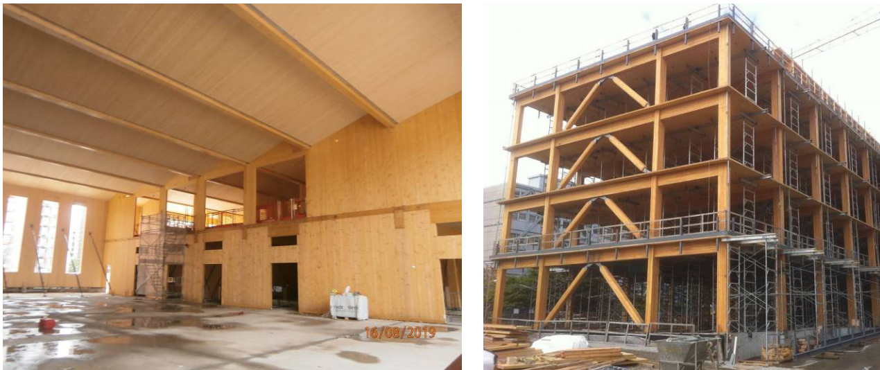
Fig. 5 – CLT building (left) and heavy timber braced frame (right – permission from Structurlam)
