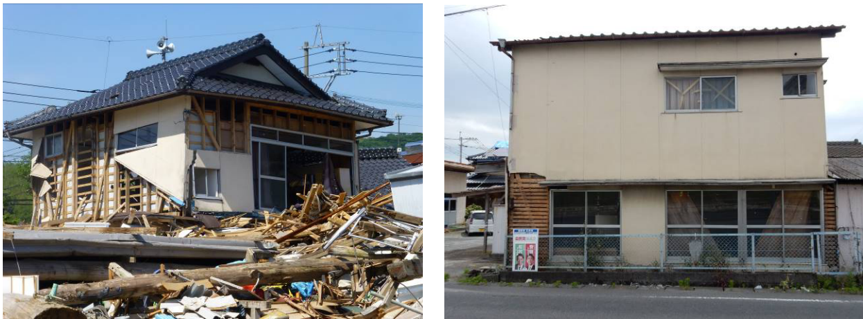
Fig. 4 – Light frame timber buildings after the 2016 Kumamoto Japan earthquake [6]
