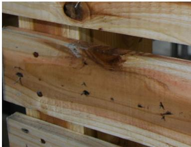
Fig. 10 - Cut staples on wooden laths
