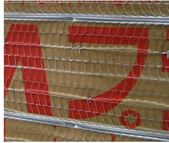
Fig. 3 - Substrate of single layer system
