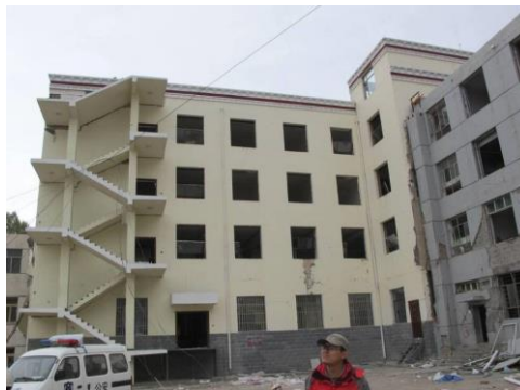
a) Overall appearance of the structure
