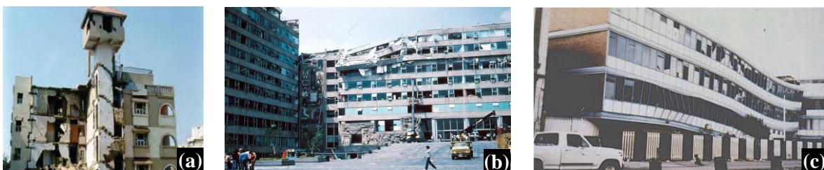
Fig. 2 – Damage observed in torsionally flexible buildings: (a) 2001 Bhuj Earthquake, (b) and (c) 1985 Mexico City Earthquake [1, 2 and 3]
