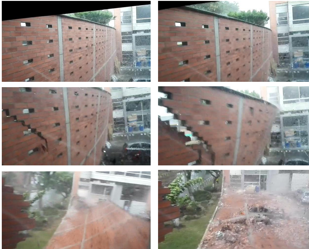
Fig. 3. – Collapse sequence obtained from video recording [1].
