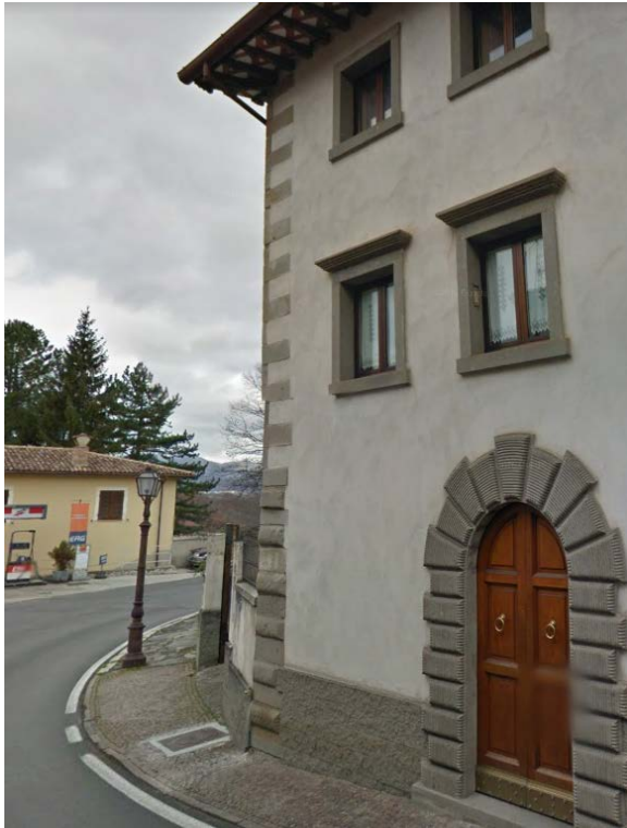
Fig. 3: Google Earth image of a building of the Amatrice historic center (left) and AEM modelling of the quoin at the masonry edges (right).
