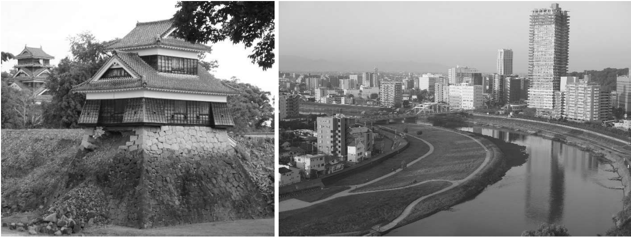
Fig. 2a (left) – Castle in Kumamoto, Japan, in 2018 showing damage from the 2016 earthquake. Damage is mostly at the top of the stone block wall; the wooden castle above does not appear damaged. Fig. 2b (right) – Urban Kumamoto, where the skyline does not exhibit gaps for collapsed or missing buildings; businesses are open and there are no signs of damage.
