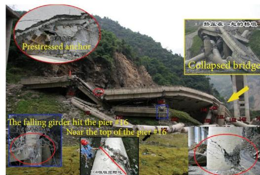
Fig. 1 - Example of bridge damage during Wenchuan earthquake
