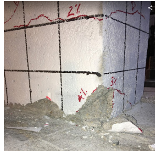
Fig. 3 – As-built wall pier spalling occurring at 4.0% drift ratio
