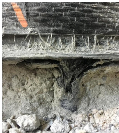
Fig. 8 – Partial anchor fracture for retrofitted wall pier with vertical CFRP anchors
