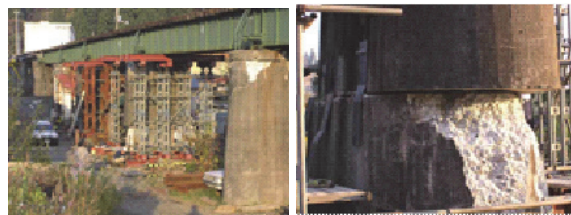
Fig. 1 – Uonogawa Bridge damaged during the 2004 Niigata-ken Chuetsu Earthquake [3]
